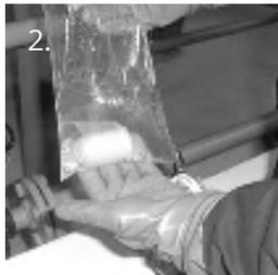
2. Unpack the Wencon Pipe Tape and submerge it in water for 10 seconds.
