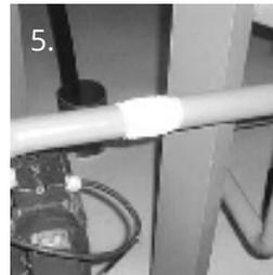
5. After 10 minutes the products semi cures, and after 60 minutes it is fully cured at 20°C (68°F).
