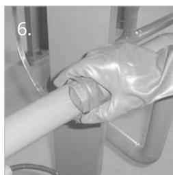
6. If the pipe cannot be emptied, use the Wencon Putty. Eventually hold it in place with a small metal plate and a steel band, before applying the pipe tape.
