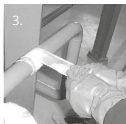
3. Wrap the Wencon Pipe Tape tight around the pipe. (min. 9 circles)
