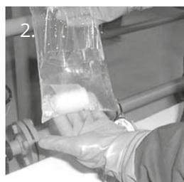
2. Unpack the Wencon Pipe Tape and submerge it in water for 30-40 seconds. For higher pressure, use Wencon Putty. (see fig. 6)
