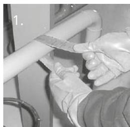
1. Empty and clean the leaking pipe and grind it with emery paper or the like. See Wencon surface preparation, next page.
